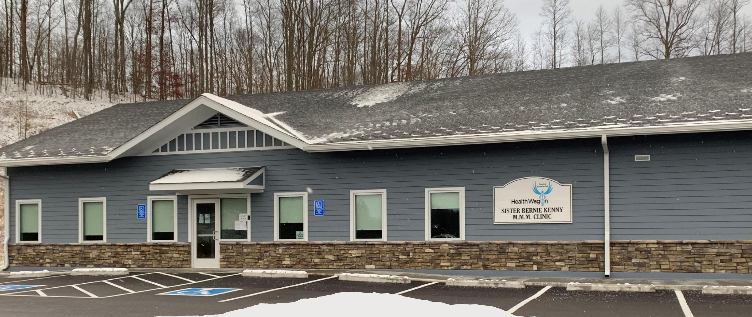
Sister Bernie M.M.M. Clinic 927 Happy Valley Drive, Clintwood, VA 24228 Built in 2020 with an Appalachian Regional Commission Grant (ARC) and Donations from Individuals and Foundations
